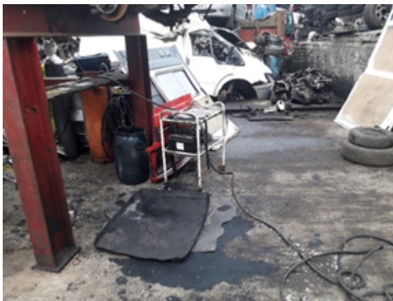
Photo Eighteen - Contaminated impermeable surface
