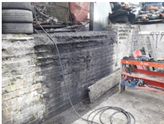
Photo Seventeen – Contaminated block wall
