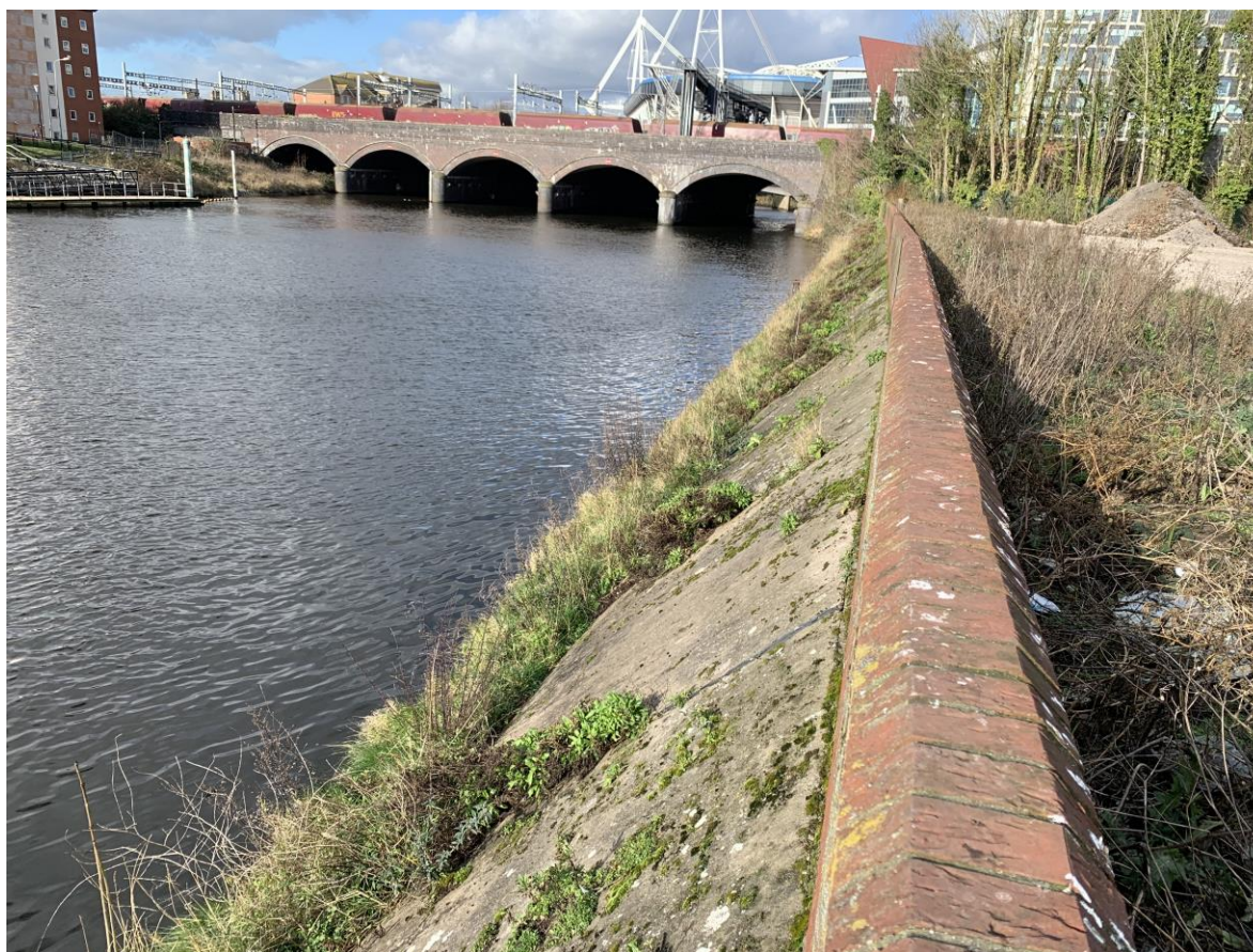
Figure 1: Existing embankment and flood wall
