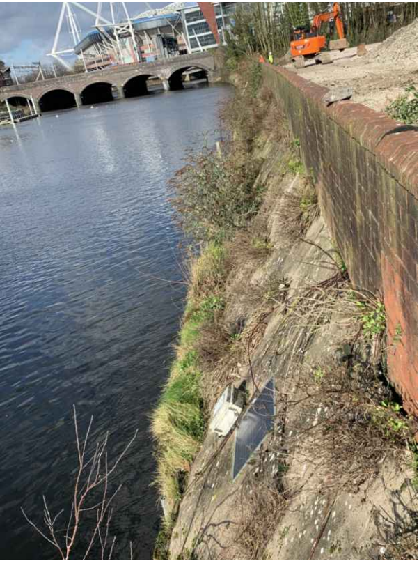
PHOTOGRAPH OF EXISTING RIVER BANK AND NRW FLOOD WALL
