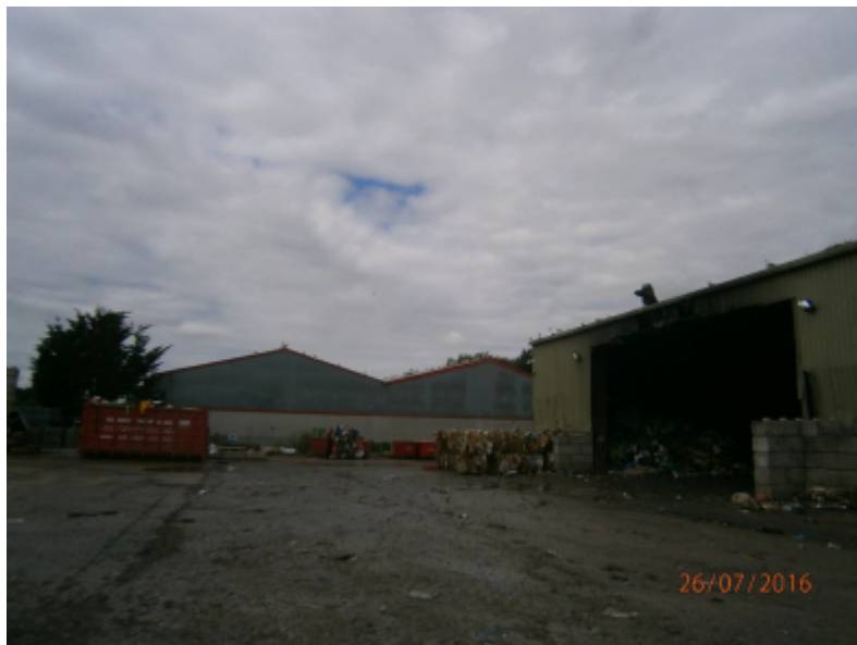
Photo 2 showing seagulls roosting on the transfer building and the neighbours building
