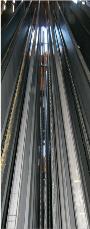
Size and soundness of electrodes as well as the pitch of channels inside the ESP allow the use of 110 kV high voltage feed
