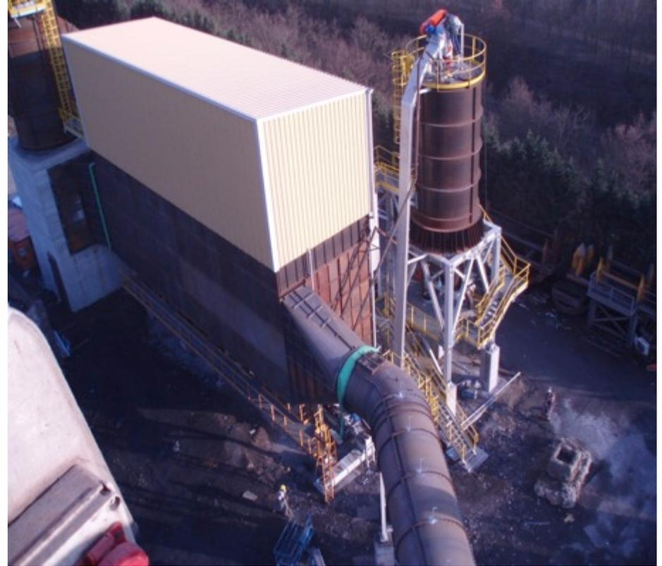
Insertion of new preseparator cyclone on dedusting plant for EAF
