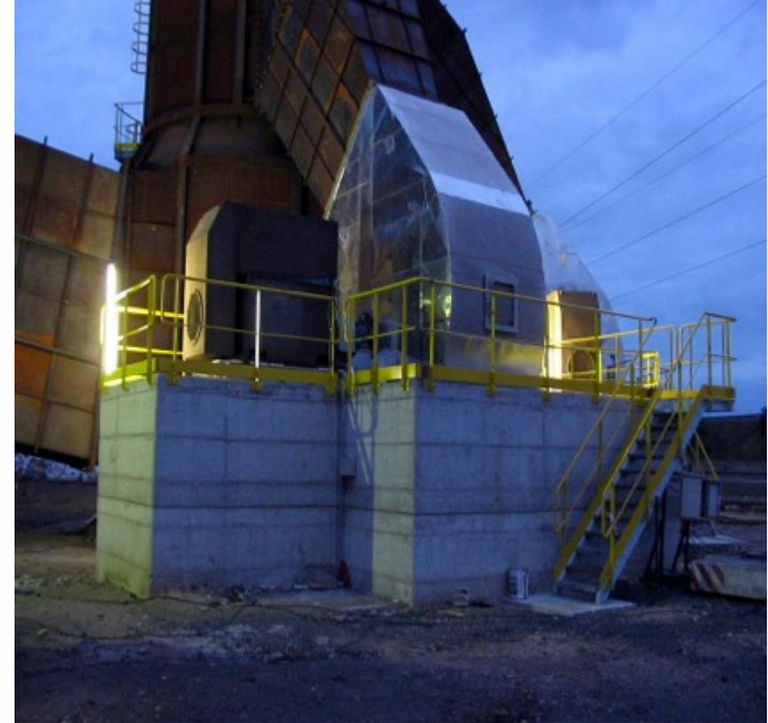
Dedusting plant with quenching tower, booster, bags filter and exhaust fans
