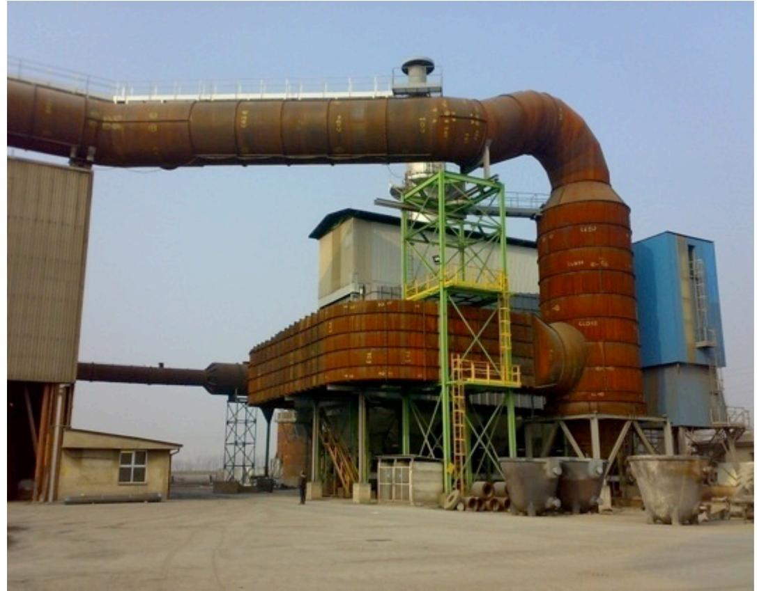
Revamping and capacity increasing of dedusting plant for EAF
