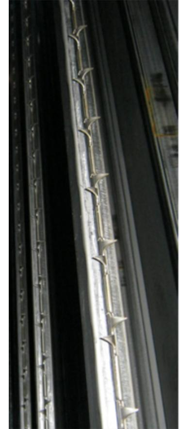
The electrodes are individually suspended at their top with the opposite end free for thermal expansion.
