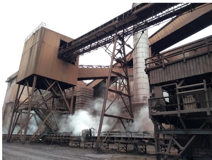
Figure A2.10 Initial site visit. Blended mix conveyor and stack
