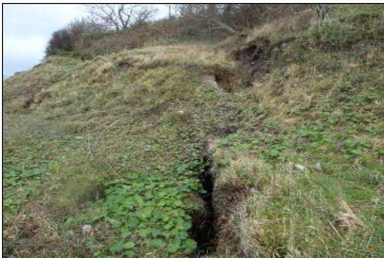
Plate 9 – Large tension crack behind slipped slope
