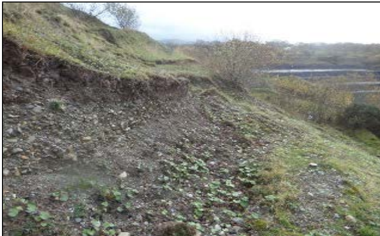
Plate 8 – Recently exposed gravel in scarp face of slipped slope
