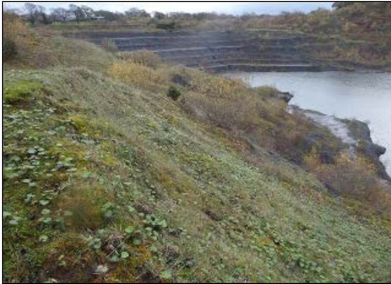
Plate 10 – Evidence of slumped soils from multiple slope failures down slope
