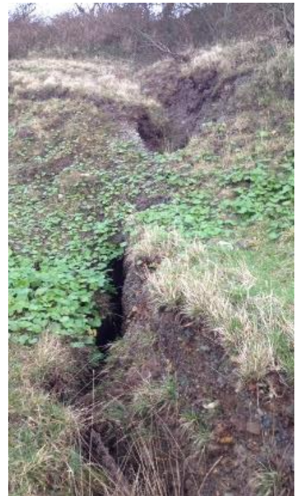
Figure 4.2: Tension crack on the eastern slopes of the quarry
