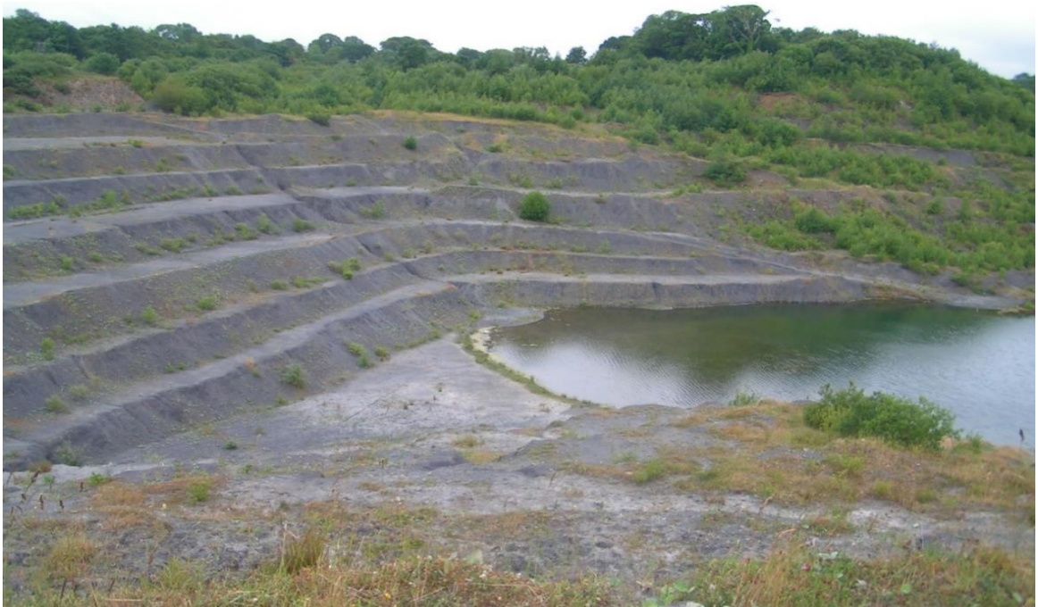
Figure 4.1: 10-year-old benches in the south face of the quarry. The foreground vegetation is a mix of annual and perennial herbaceous plants growing on bare, weathered overburden, while growth on the benches (left) only occurs in accumulated wash-off from the steep slopes. The background slopes to the right have been formed without benches and are developing woodland cover on very old weathered clay and overburden. The trees on the upper quarry slopes are on overburdens that have been exposed to weathering for in excess of 16 years.
