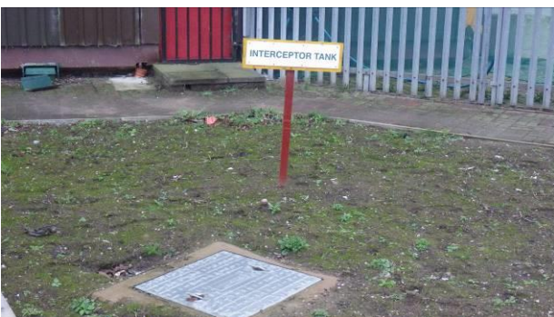
Photograph 14. Location of interceptor tank.
