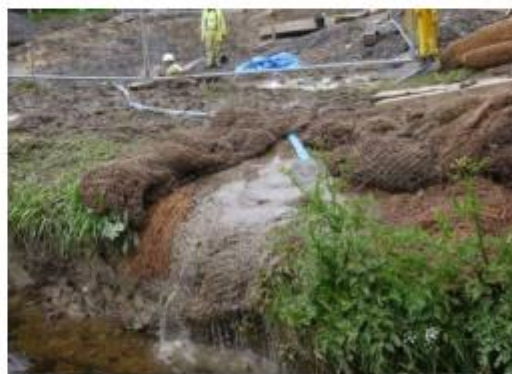
Deployed to treat muddy excavation water
