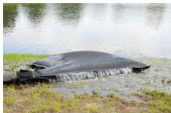
Cut open bag to show trapped silt
