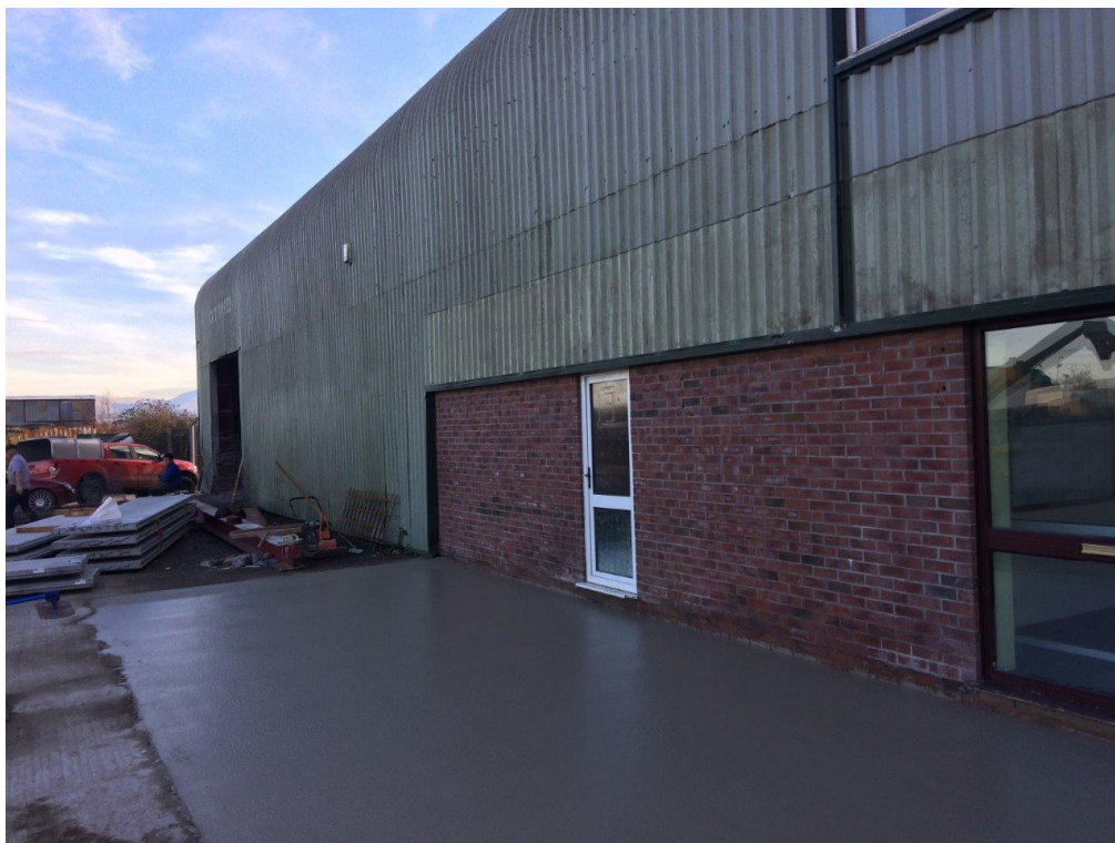
Photograph 4: New concrete surfacing on the north side of the new transfer building
