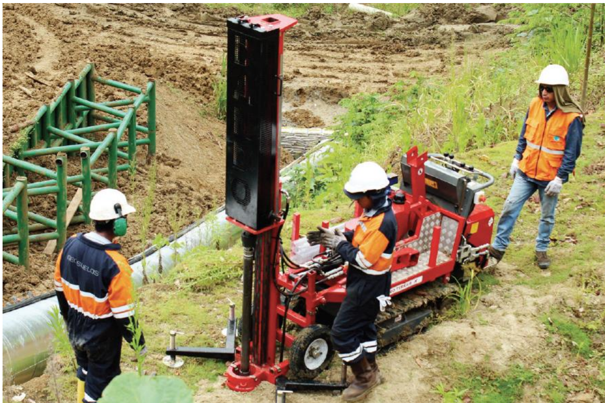
Terrier Rig tracked boring rig
