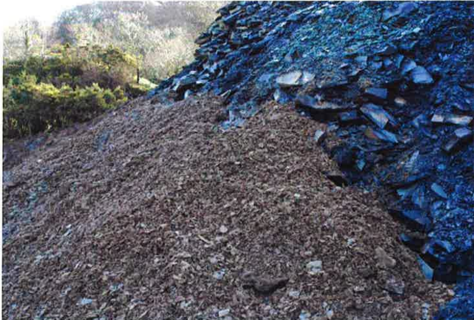
Plate 1: Waste arising from slate waste reprocessing operations at Ty Mawr West Quarry generally containing soil-forming materials placed against existing tipped slate waste as part of restoration (February 2012).
