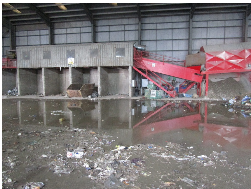
Figure 5. Wastewater from the fire contained inside the building.
