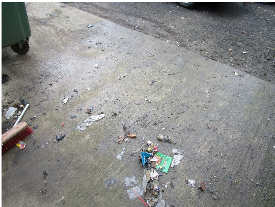
Figure 6. Waste and water marks beyond the interceptor drain showing the wastewater by-passed the drain.
