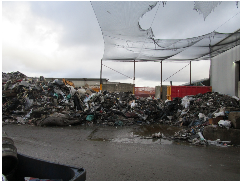
Figure 2. Mixed waste pile where the fire incident occurred. Fire break walls surrounding the waste pile and between the waste and the outbuilding.
