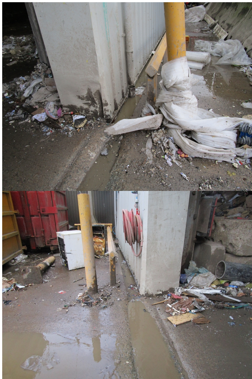
Figure 3. Site culverts that captured the wastewater directly from the mixed waste pile
