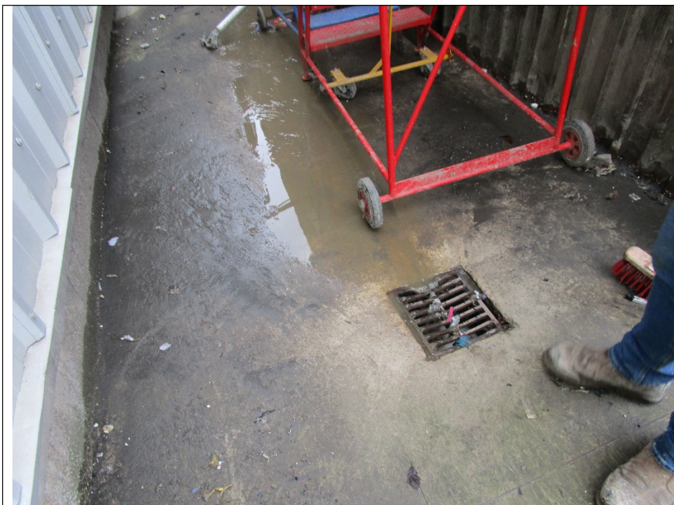
Figure 4. Discharge into the site's interceptor from the site's culverts.
