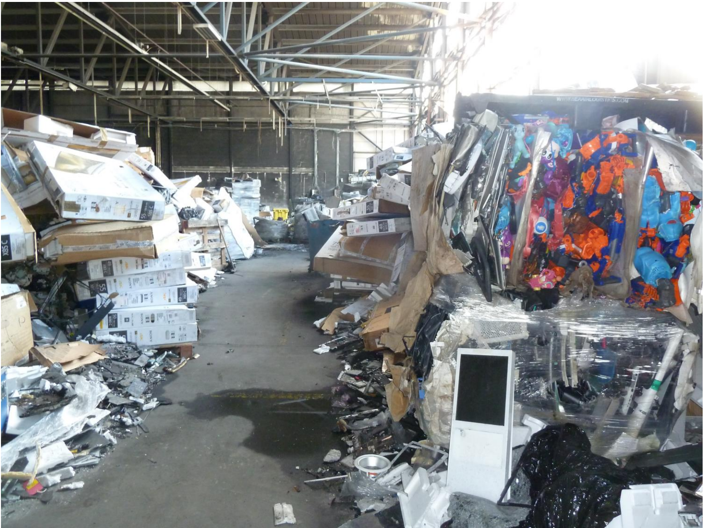
Photograph showing waste stored inside damaged building (Photo ref P1020350)
