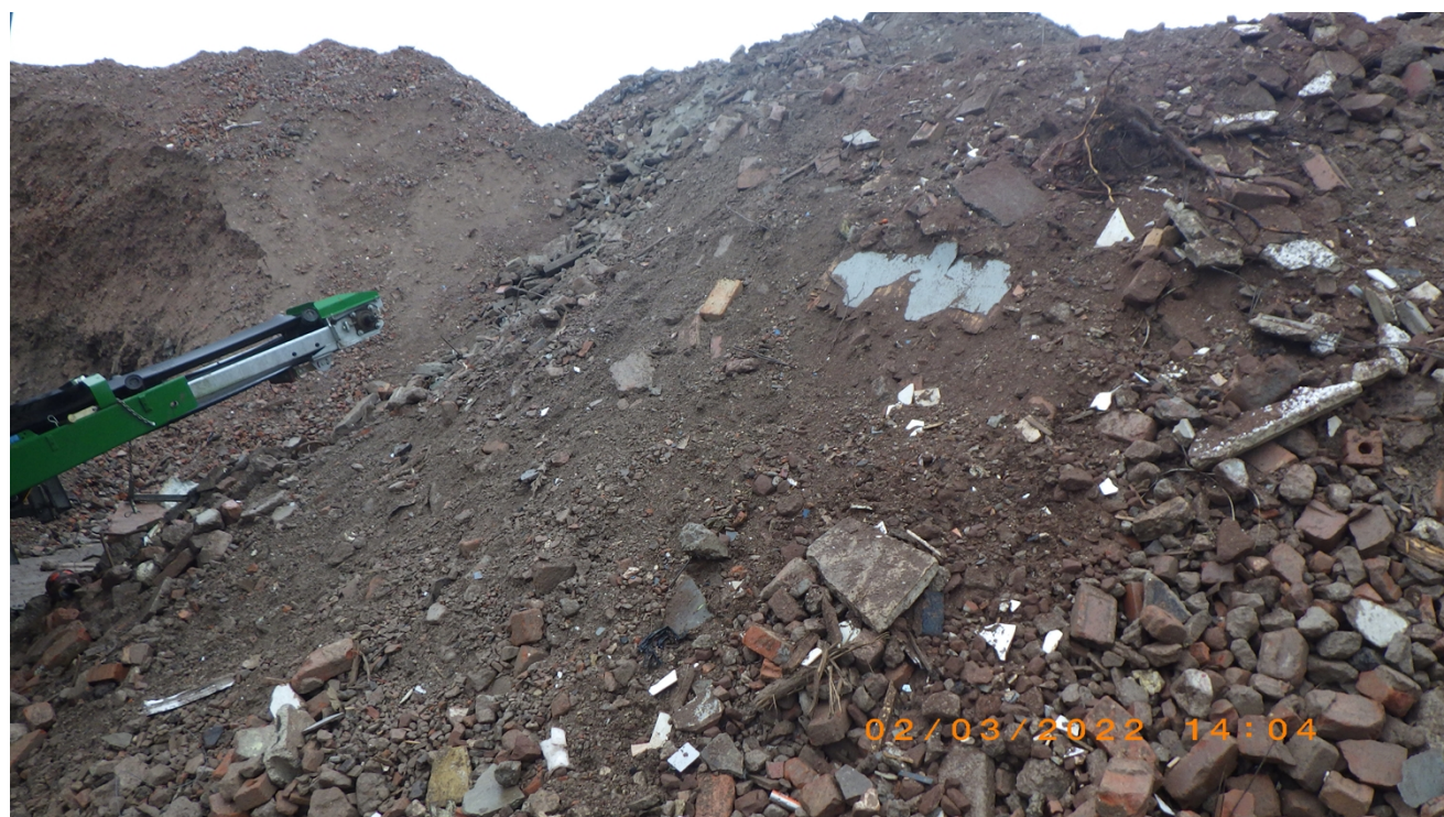
2) Photograph showing storage of inert wastes adjacent to finished product
