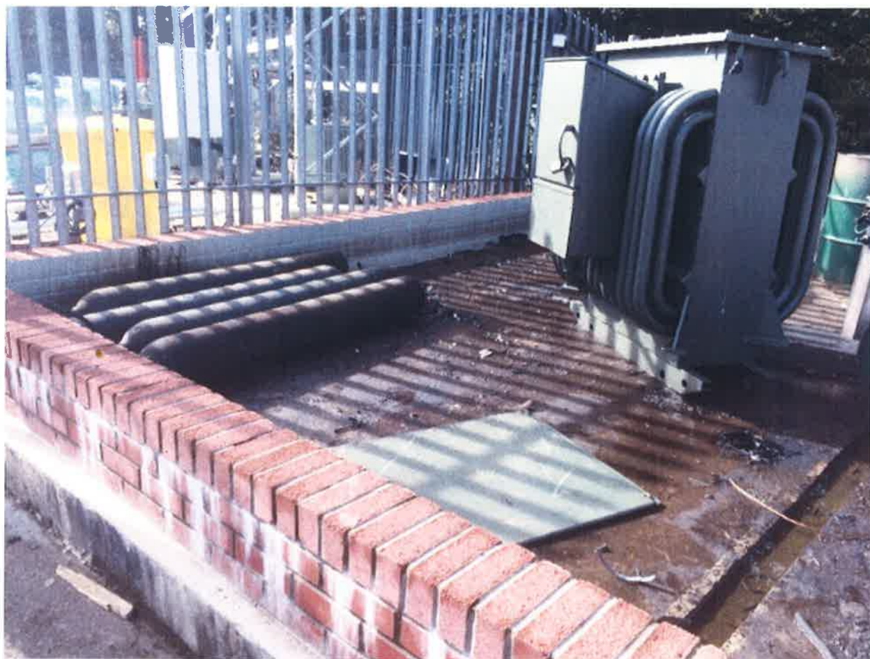
Picture 1 – redundant transformer bund
