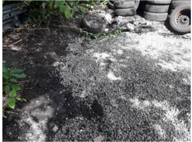
Photo Four – Hardstanding surface
