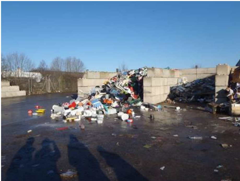
Image 1 – Newly installed concrete bays for waste stream separation.
