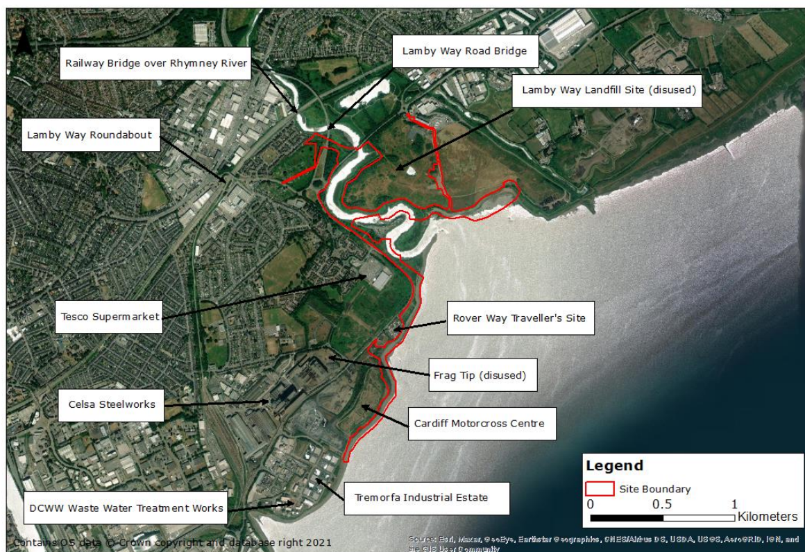
Figure 2-2 Aerial imagery of the development site and surrounding area
