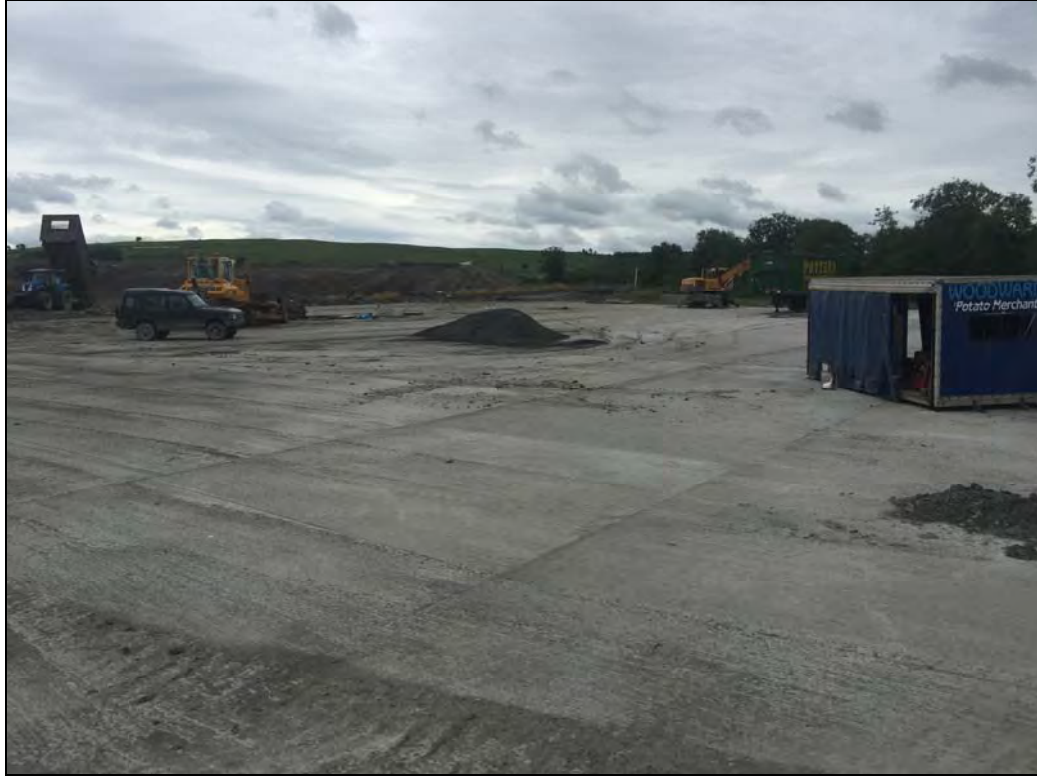
Figure 10: Compost pad concrete slab completed
