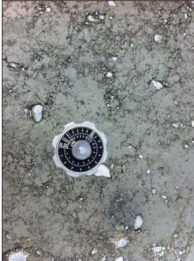
Figure 2: View of shear vane test carried out on sub grade formation pre concrete placement
