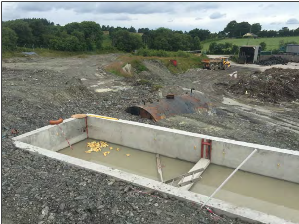
Figure 8: View of settlement pit and holding tank
