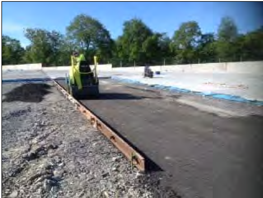
Figure 3: Compaction of sub base pre placement of concrete
