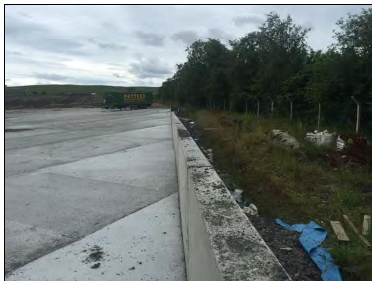
Figure 6: View of western concrete wall
