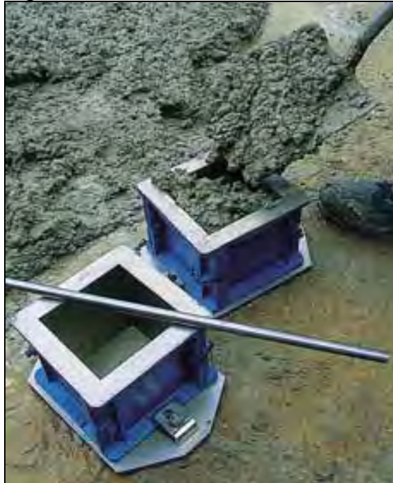
Figure 5: Cube test taken on site in 2016
