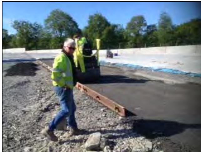
Figure 4:100mm steel shuttering
