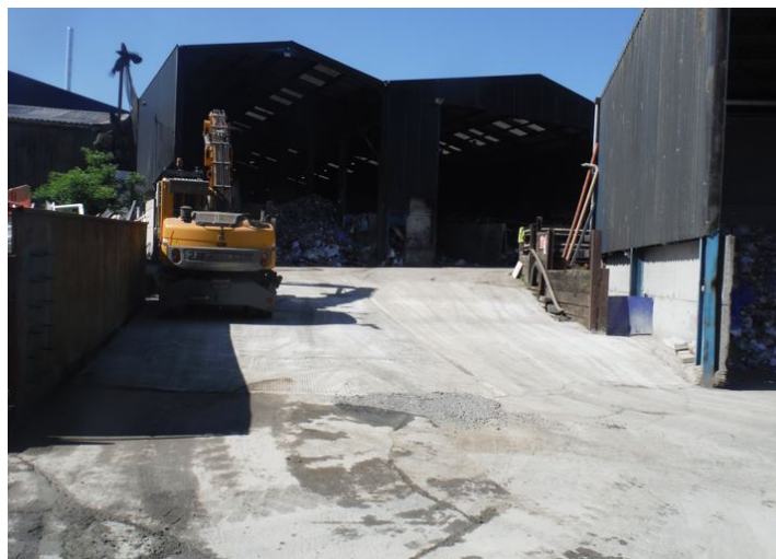
Photo 2: New ramp near the Materials Recycling building.
