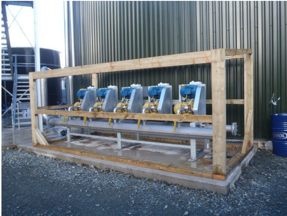
Frame for acoustic cladding around compressor pumps
