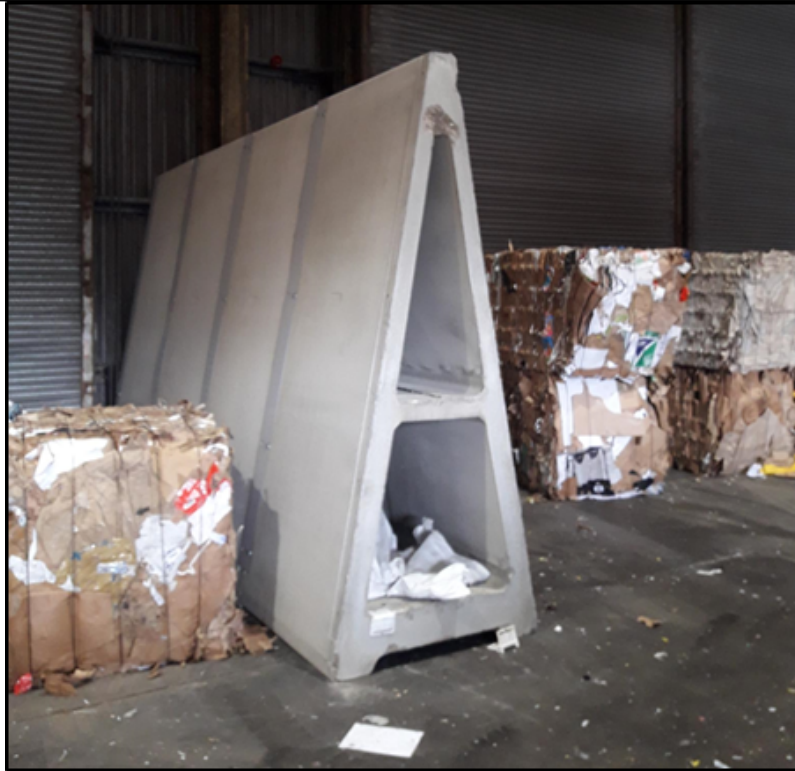
Image 1 – showing a fire wall separating baled materials
