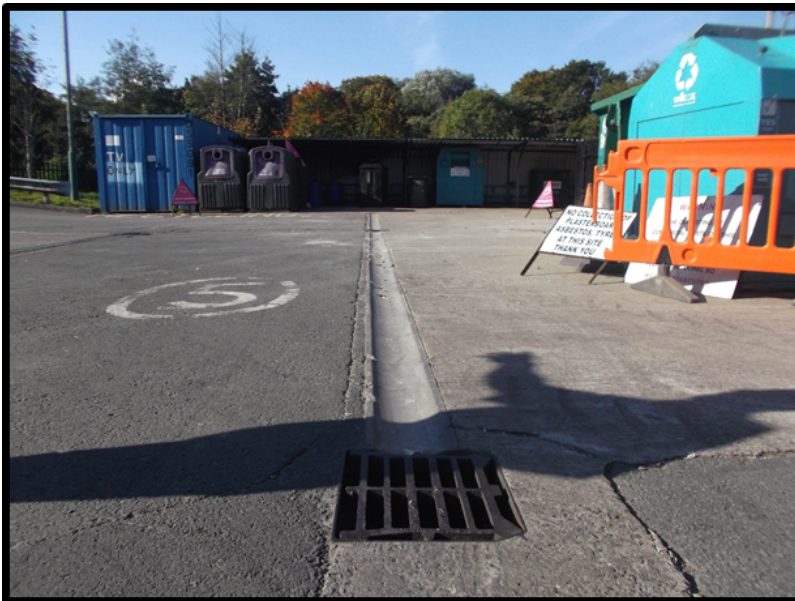
Picture 1 – showing the channels that lead to the drains installed about three years ago; no apparent issues.
