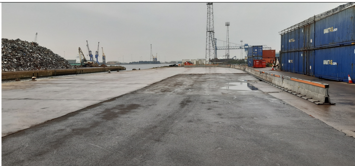
Photo 1 - ABP Site, Newport
