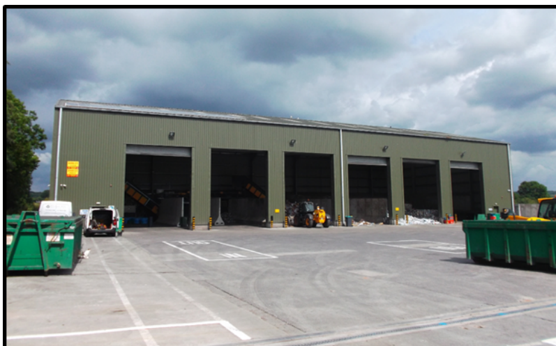
Picture 1 - Showing unit covering material sorter and separated waste bays
