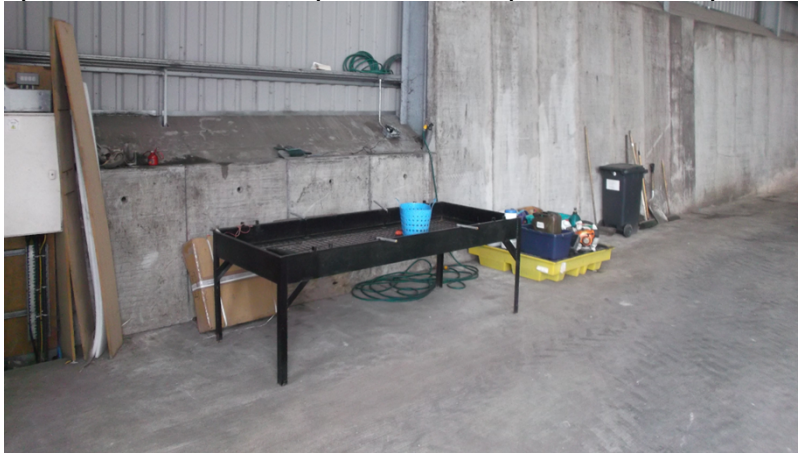
Picture 2 - showing sampling station and stored chemicals on impermeable pad
