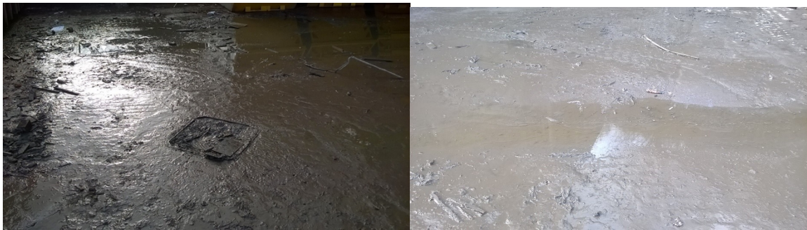
Picture showing gully leading to the interceptor Picture showing interceptor drain at bottom of site
