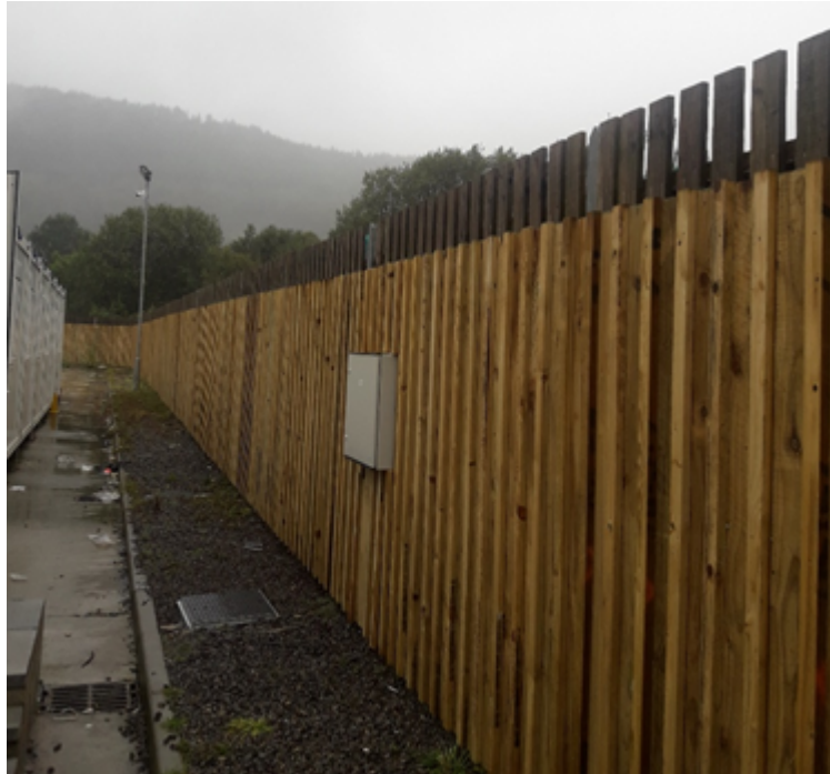
Figure 1 – additional layer of timber applied to acoustic barrier
