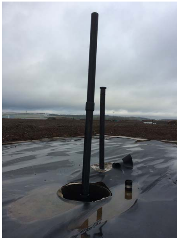
Plate 4. Construction of Gas Vents through Capping Systems
