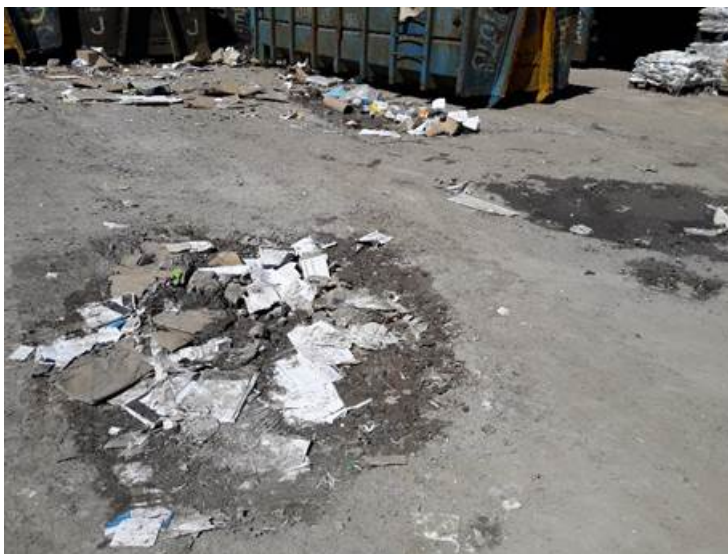
Picture 2: Rutting and surface damage
