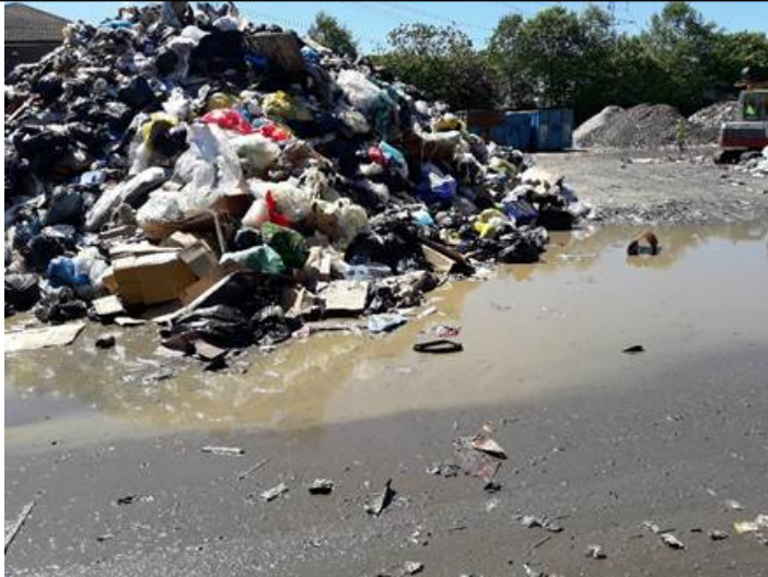
Picture 1: Blocked drain
