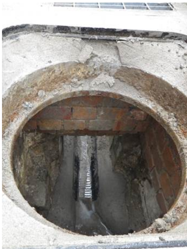
Photo 2: Newly installed drains to improve flow and avoid stagnant pools
