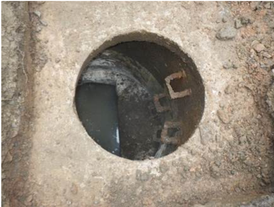
Photo 3: E9 chamber following improvement work
